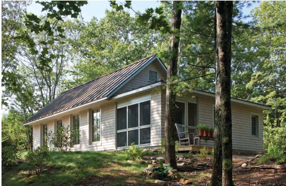
Site sensitive. Placing the house in a small clearing preserves aspects of the site that made it an attractive place to build. Cedar shingles and a metal roof are durable and low maintenance, and complement the setting. Photos left and above taken at A and B on floor plan, respectively.
