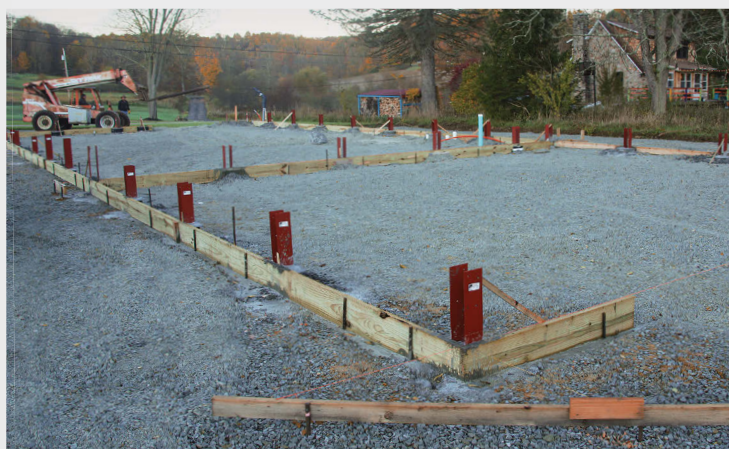
Set the post brackets. The brackets that attach the posts to the concrete piers are wet-set into the concrete and aligned to stringlines indicating the building footprint. Setting up the strings correctly and placing the post bases accurately is crucial for getting a straight, square building.
